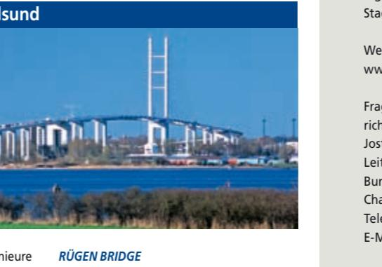
innovations into the construction of the Rügen Bridge. For the first time in Germany, they used interlaced cables (multiple layers of intertwined round wire) as design elements. The pylons and all abutments are built in the shape of a teardrop. They used self-compacting concrete in the Y-support connection zones. They also used a wind-deflecting design for the guardrail cladding and increased the safety standards of the protection system.
